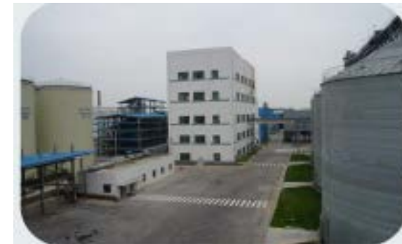
Dongguan, Guangdong, China – Oilseeds crushing plant
